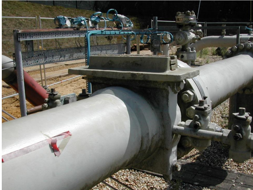
Figure 4.2 – Daniel Orifice Fitting
