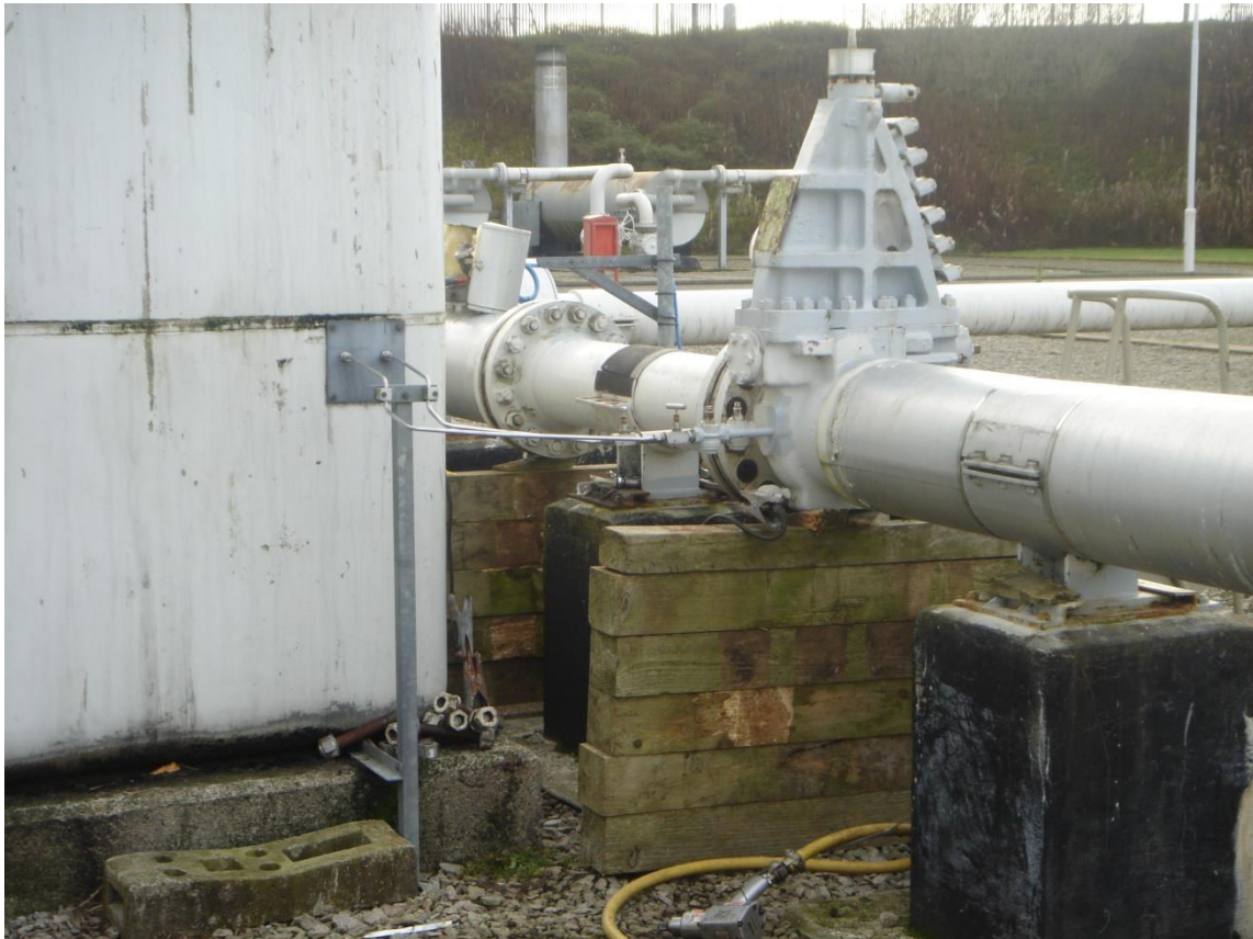
Figure 4.4 – Downstream Pipe Section
