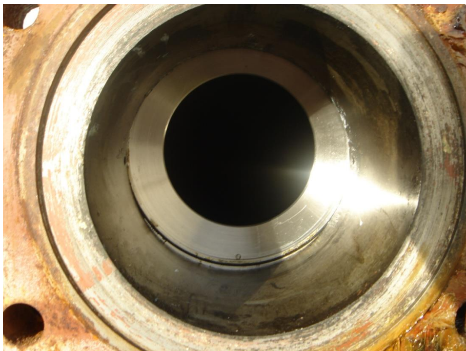
Figure 5.2.2 – Orifice Plate Position (Counter Reading 99995)
