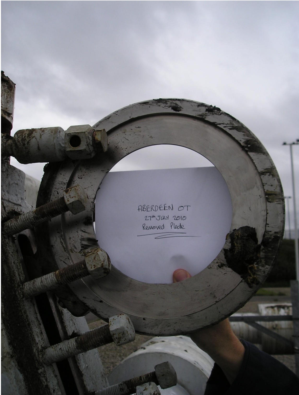
Figure D.2 – Orifice Plate (“As Found”) 27 th July 2010
