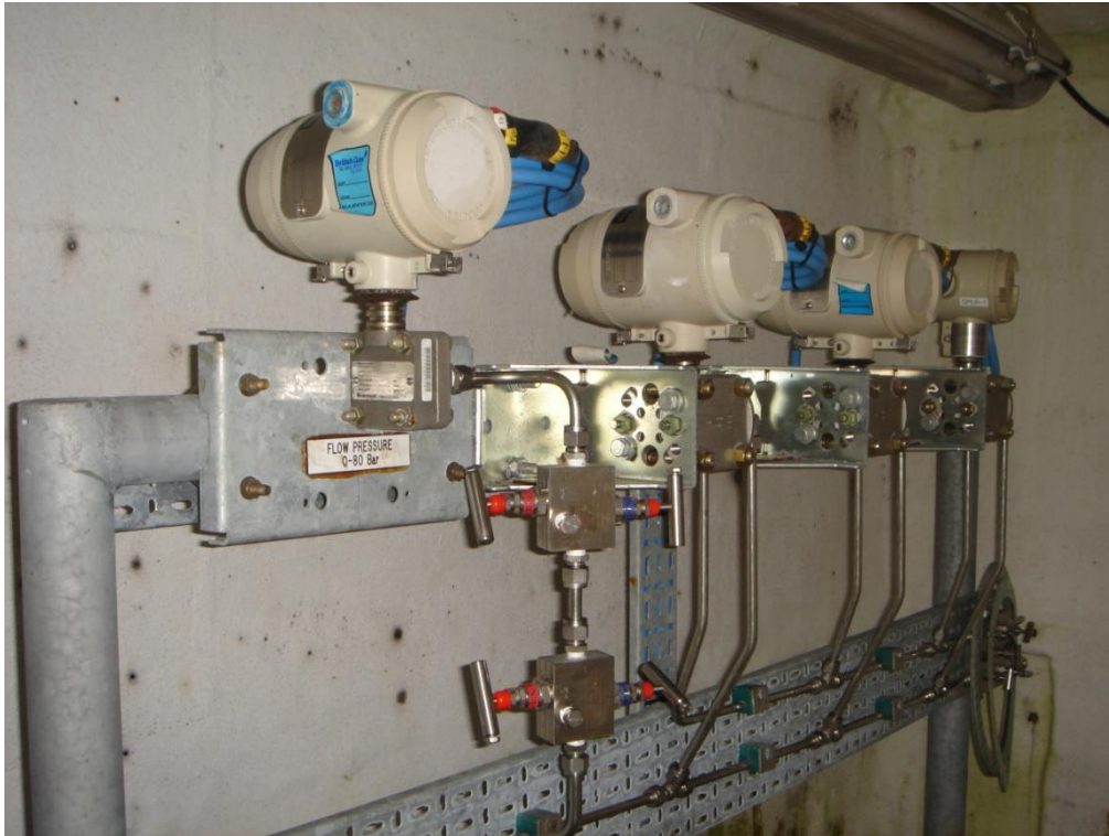
Figure 4.5 – Transmitter Mounting Rack
