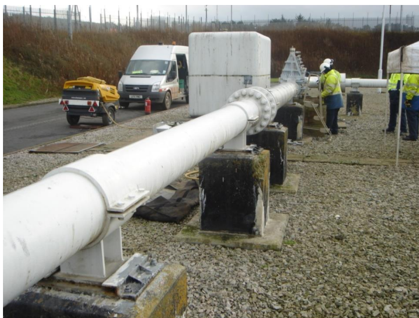
Figure 4.3 – Upstream Pipe Section
