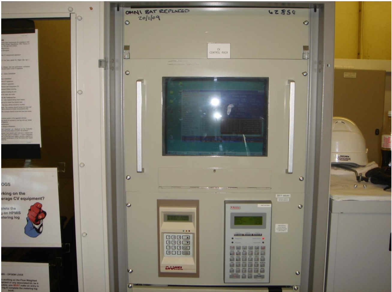
Figure 4.7 – Metering Panel
