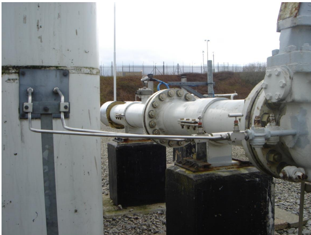
Figure 4.6 – Transmitter Impulse Lines
