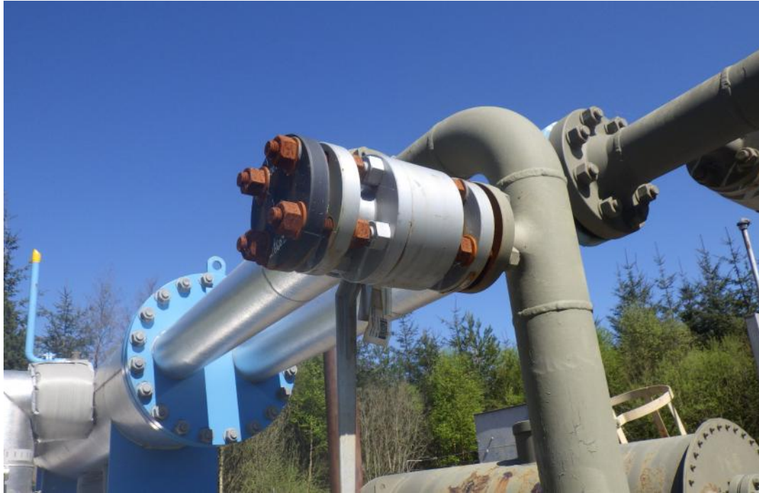
Figure 4: Pro-Heat Immersion Tube Preheater at Lochmaben (Existing Water Bath Heater in background)
