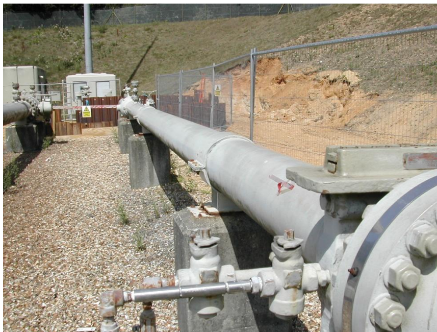
Figure 4.3 – Upstream Pipe Section
