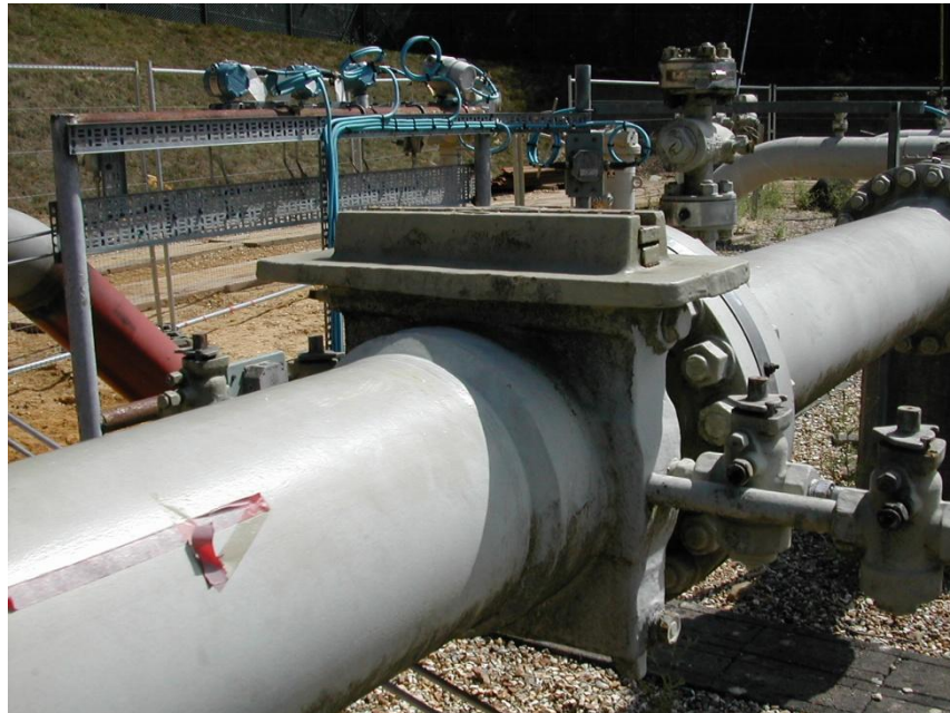
Figure 4.2 – Daniel Orifice Fitting
