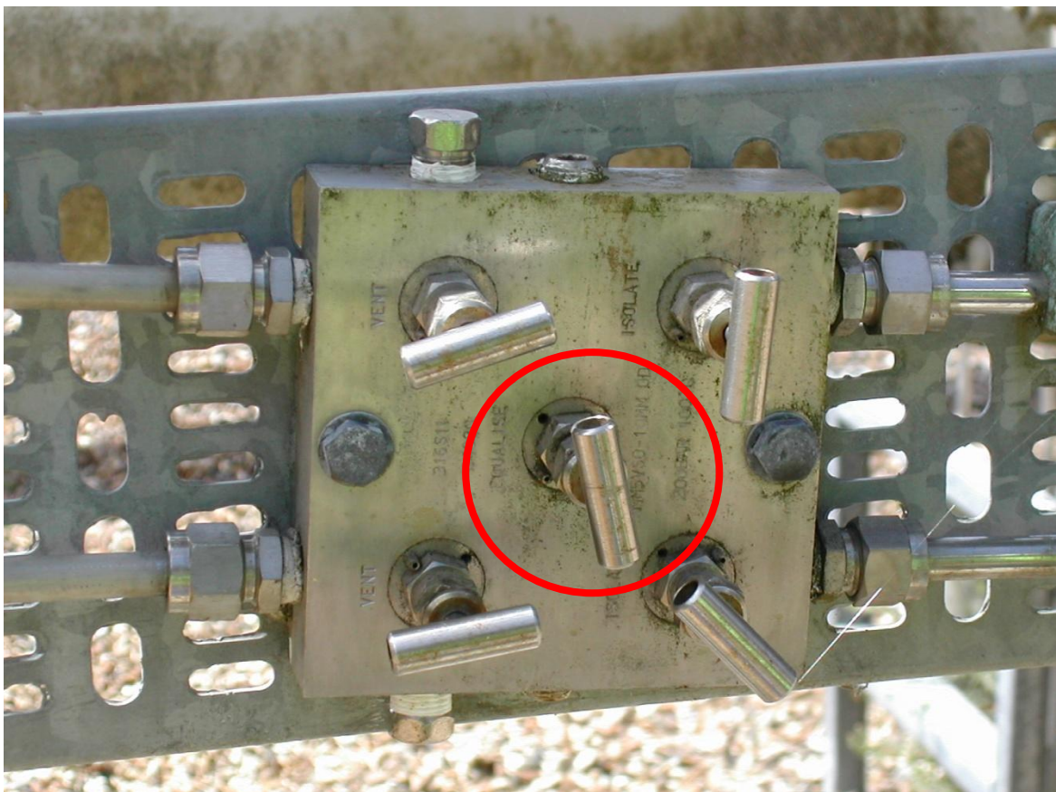
Figure 3.4 – Common \Delta P Isolation Manifold
