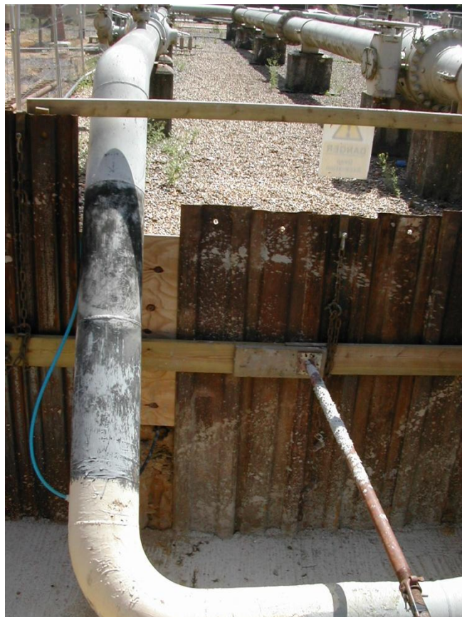
Figure 4.5 – Normally Buried Inlet Section
